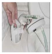
Push float box completely down, between the two ribs.
